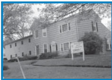
The Fayette County Health Department is housed in this 100-year old building on 509 West Edwards Street, Vandalia, Illinois.
